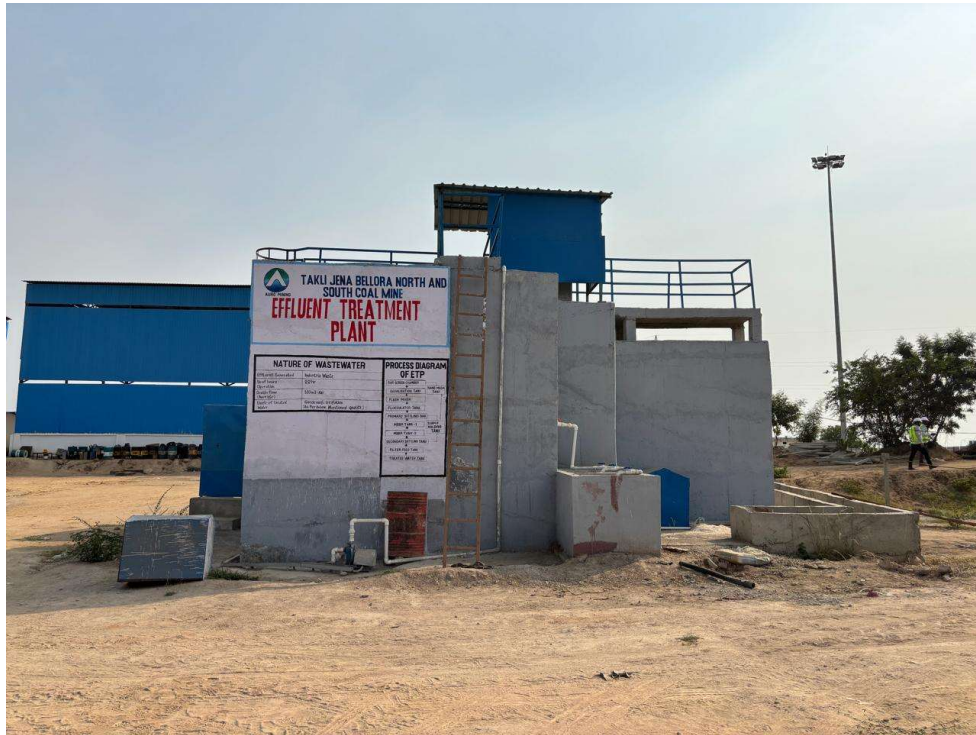
ETP of 100 KLD ready for operation
