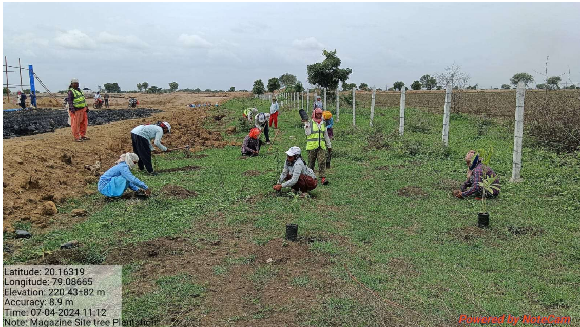
Plantation conducted near new coal stock area
