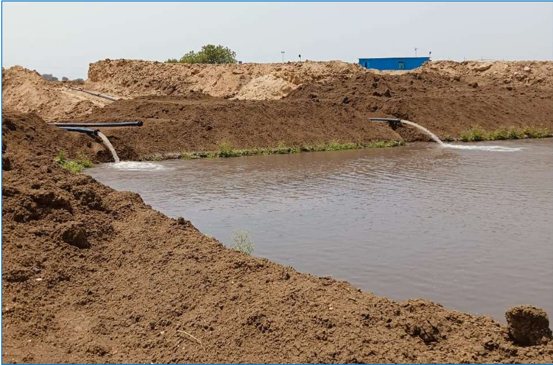
Mine seepage water pumping into sedimentation tanks
