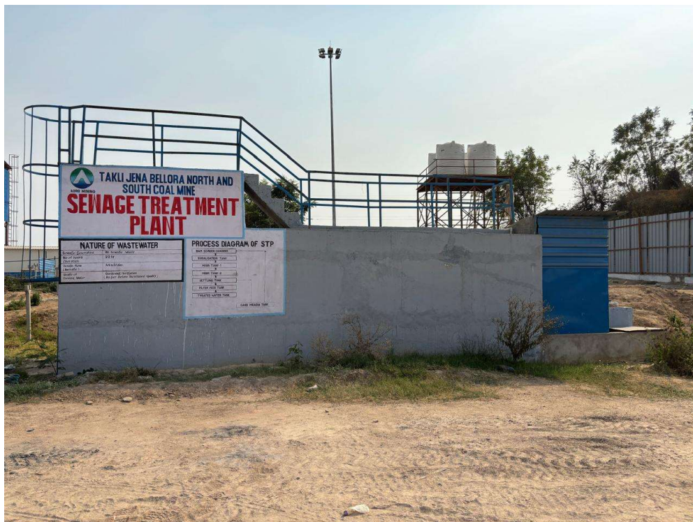
STP of 44 KLD ready for operation
