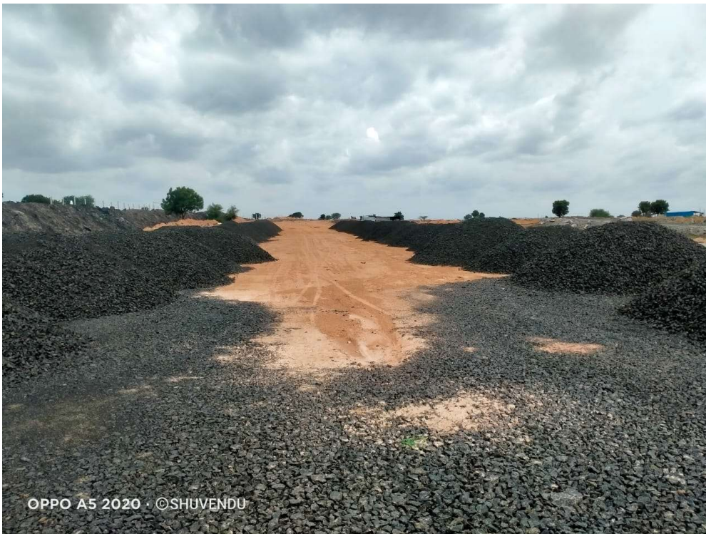
Transportation road work in progress
