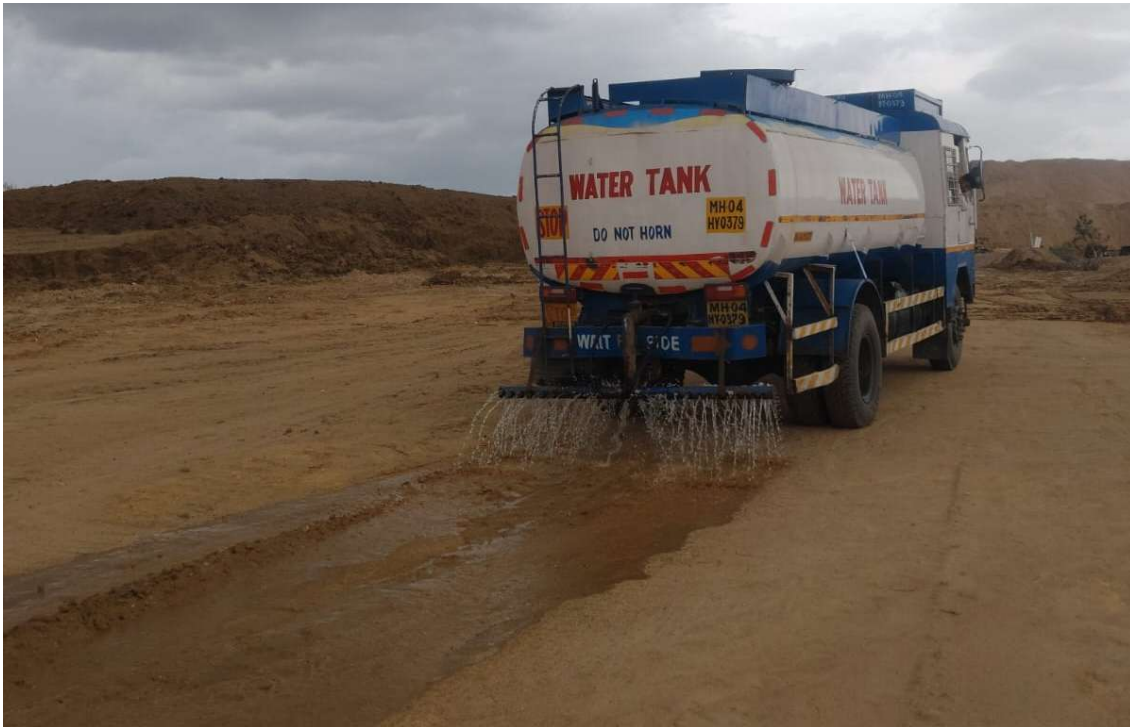
Water Sprinkling on Haul Road
