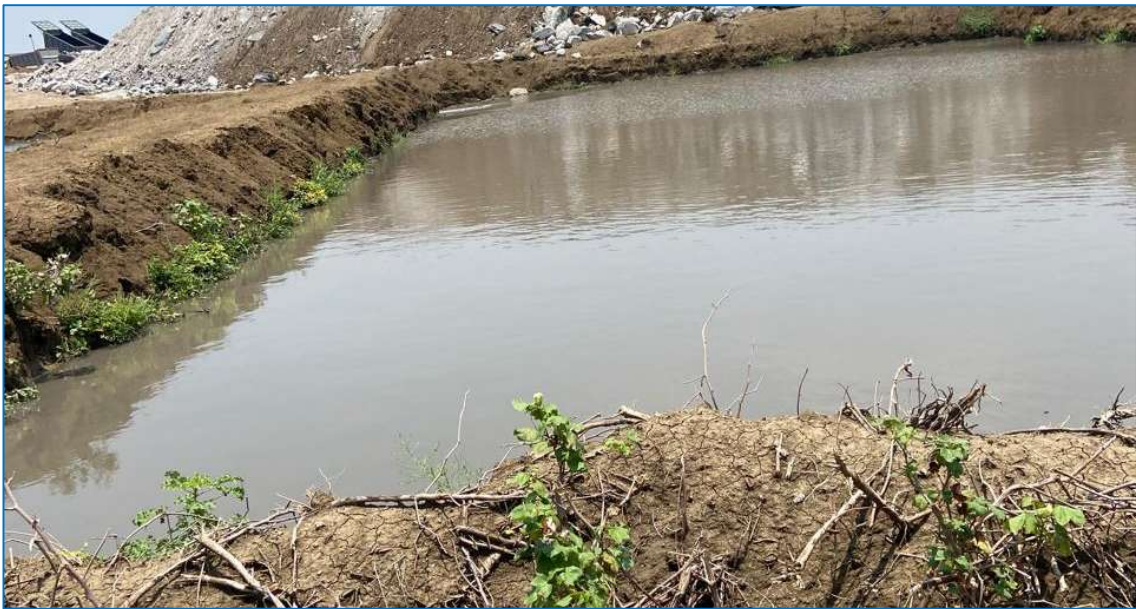
Series of Sedimentation tanks (3 no's)
