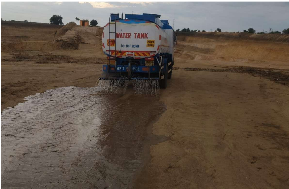
Water Sprinkling on haul road
