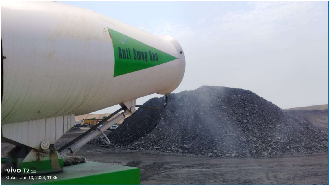
Fog Canon arranged at haul road
