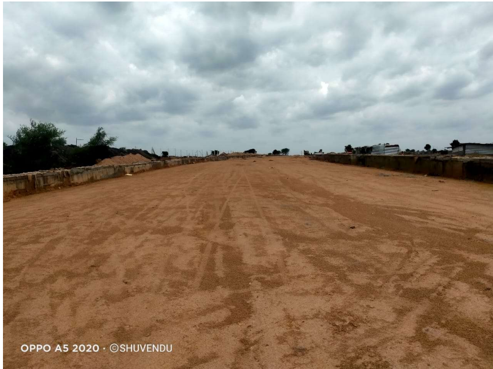
Transportation road work with side drains
