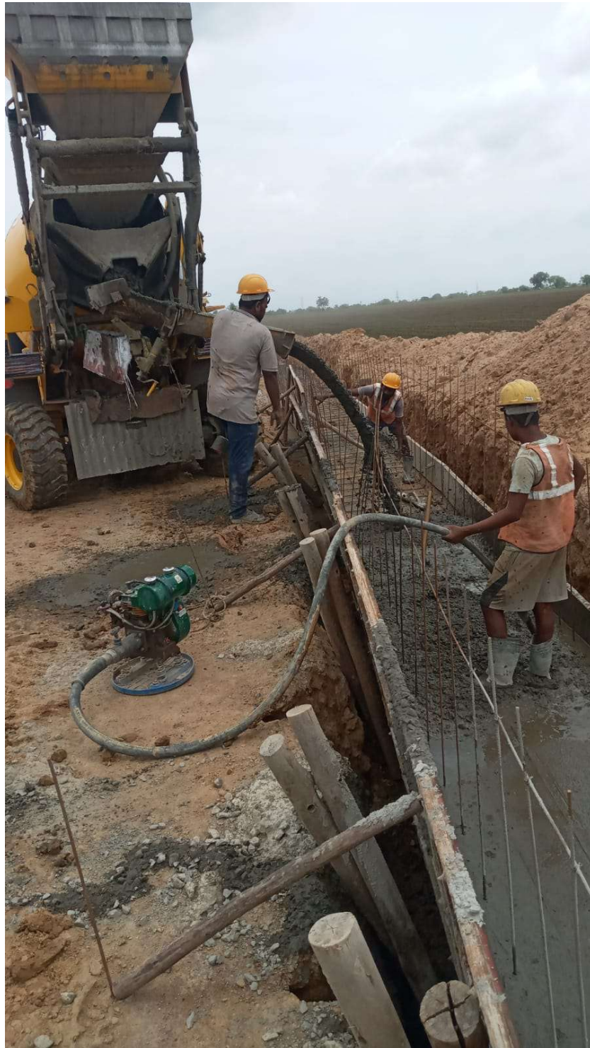
Annexure - 8 – Coal transportation road work in progress
