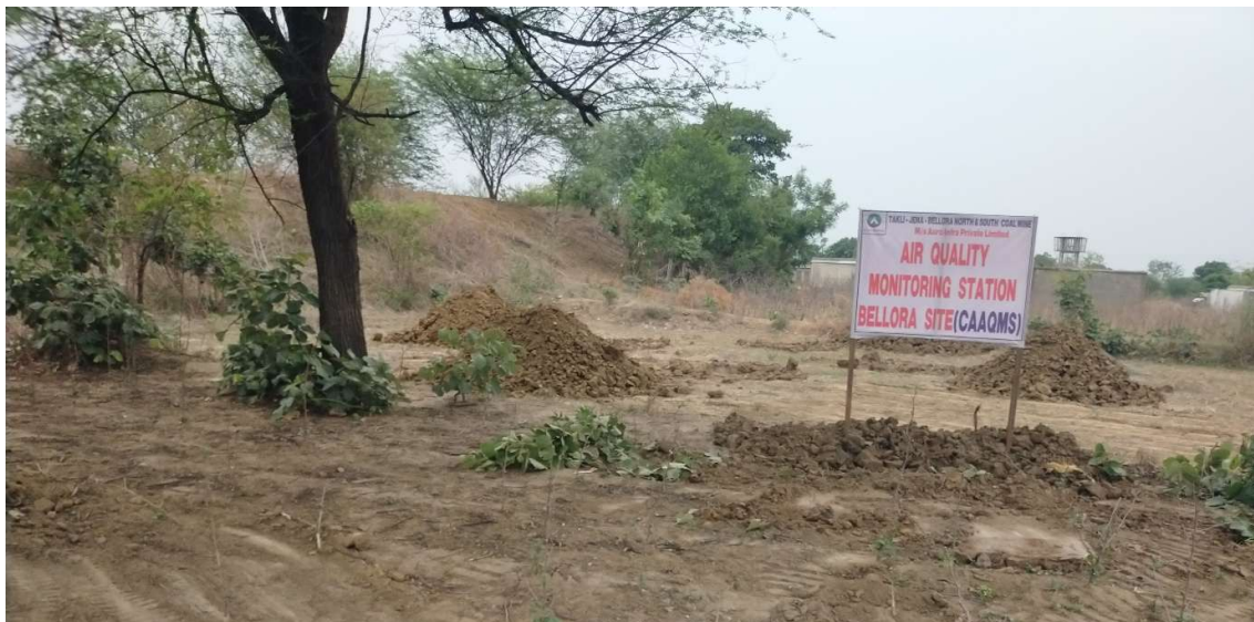
2. CAAQMS under installation
