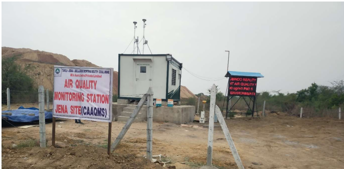
1. CAAQMS under operation
