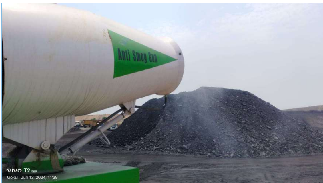
Fog Canon arranged at haul road
