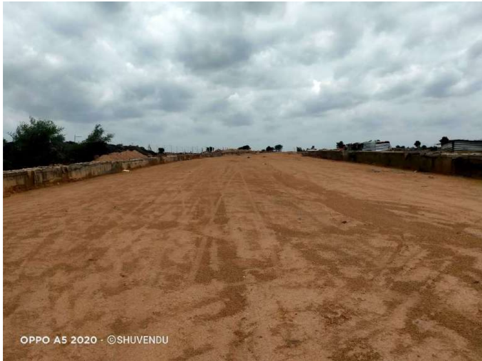
Transportation road work with side drains
