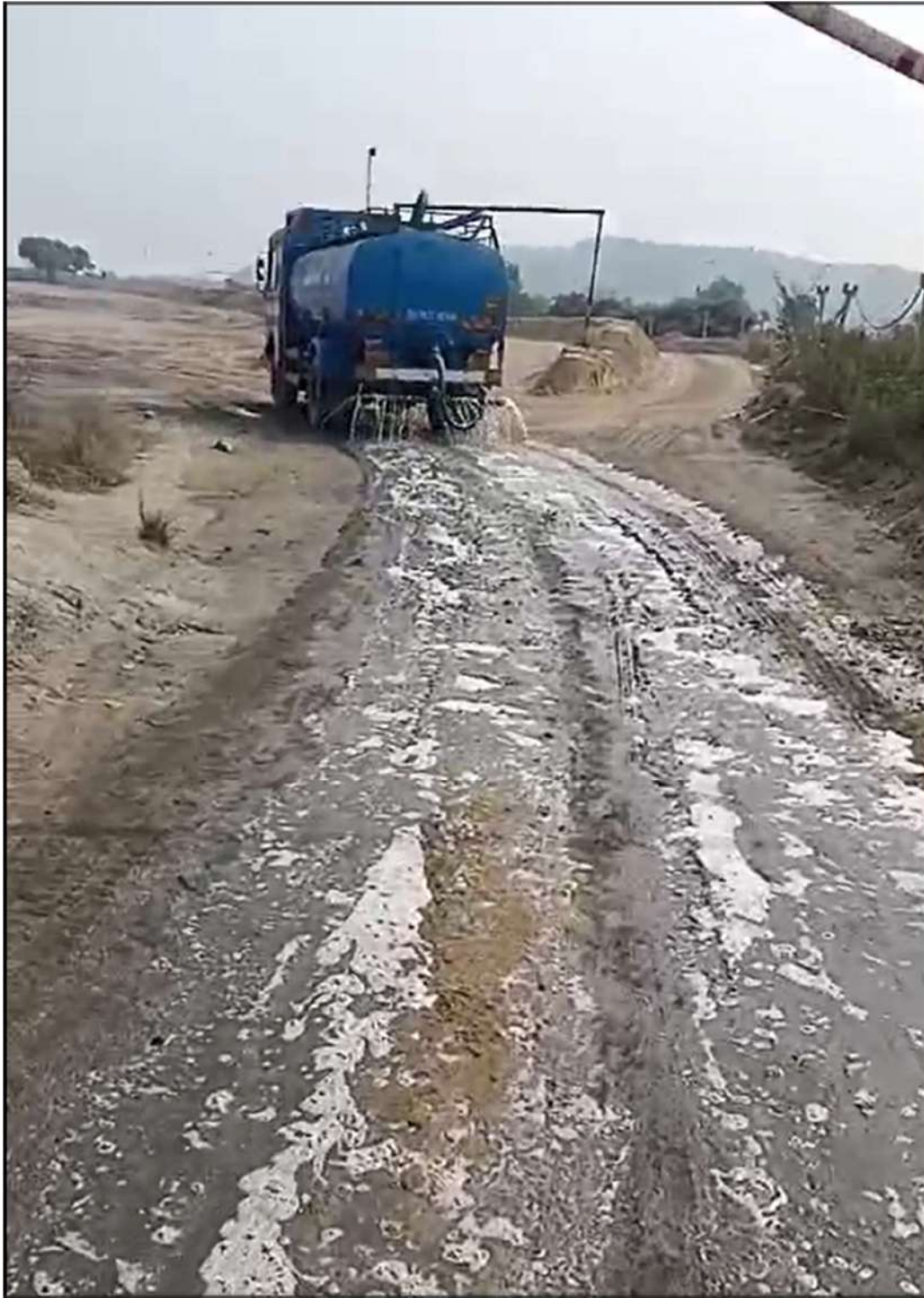
2. Water sprinkling on haul road near Coal stock yard (12KL)
