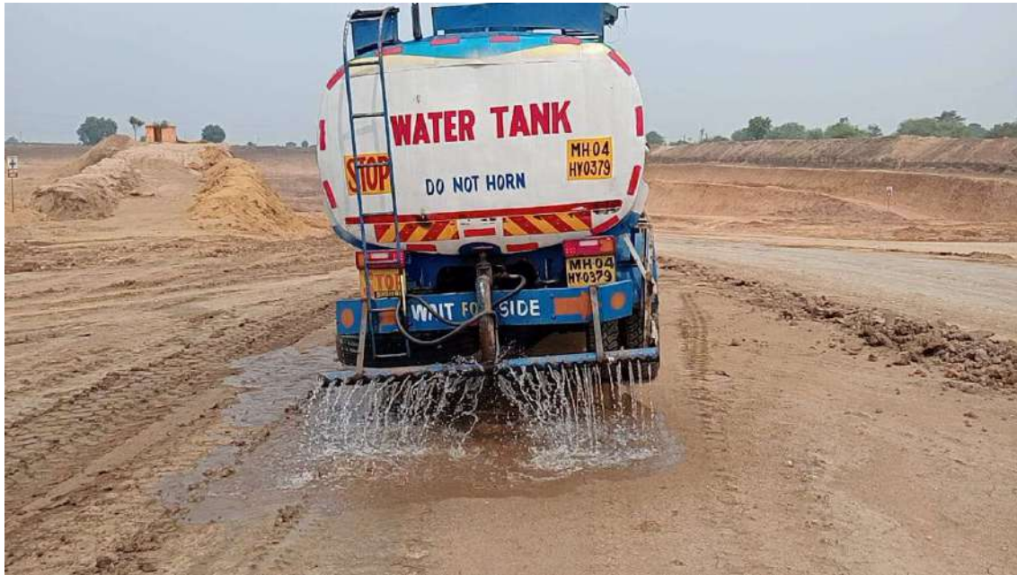
3. Water sprinkling on near OB dump (12 KL)
