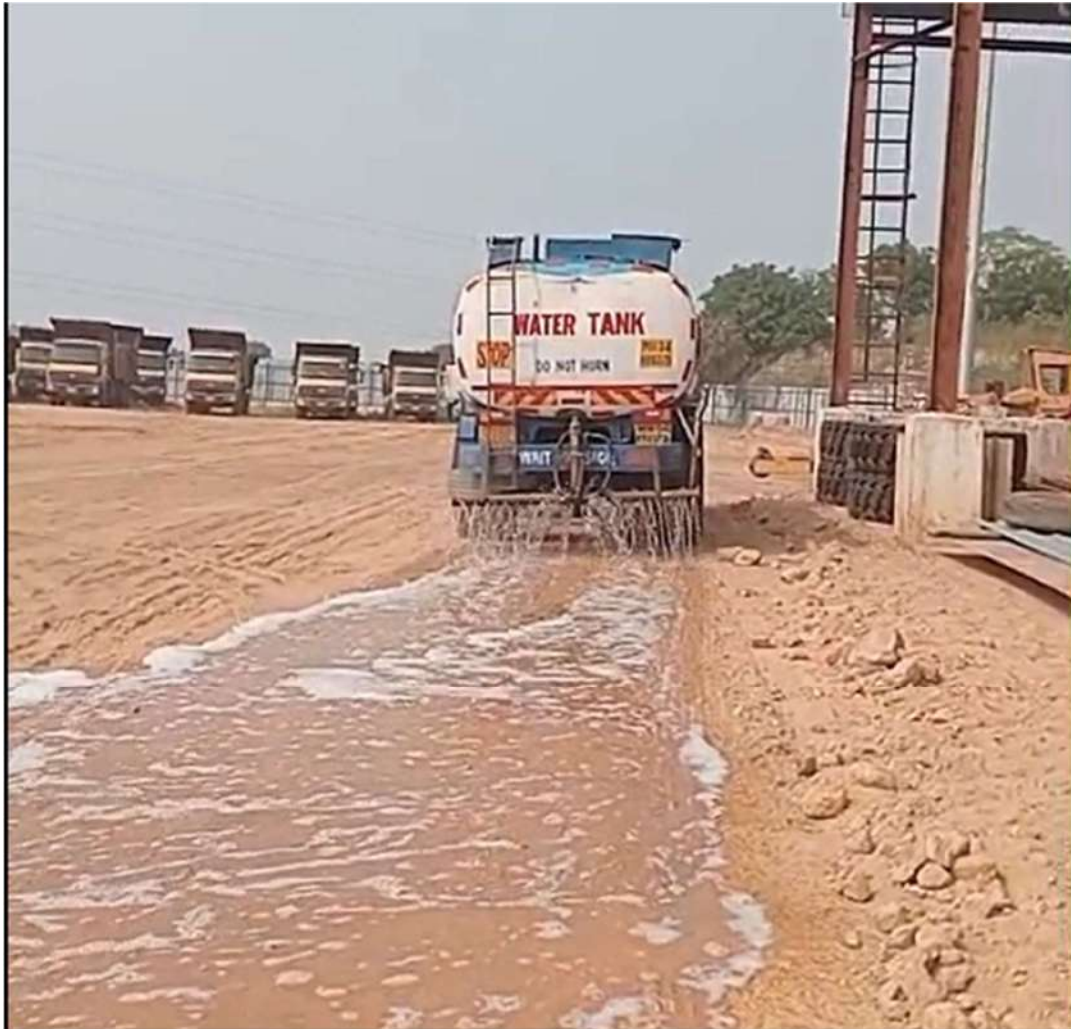
1. Water Sprinkling near workshop area (12KL)
