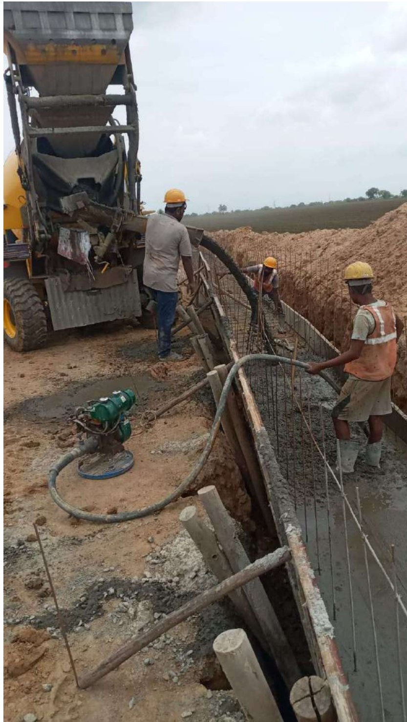
Annexure - 8 – Coal transportation road work in progress
