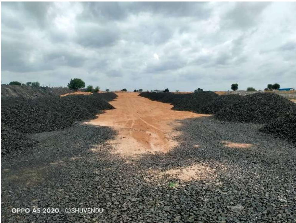
Transportation road work in progress
