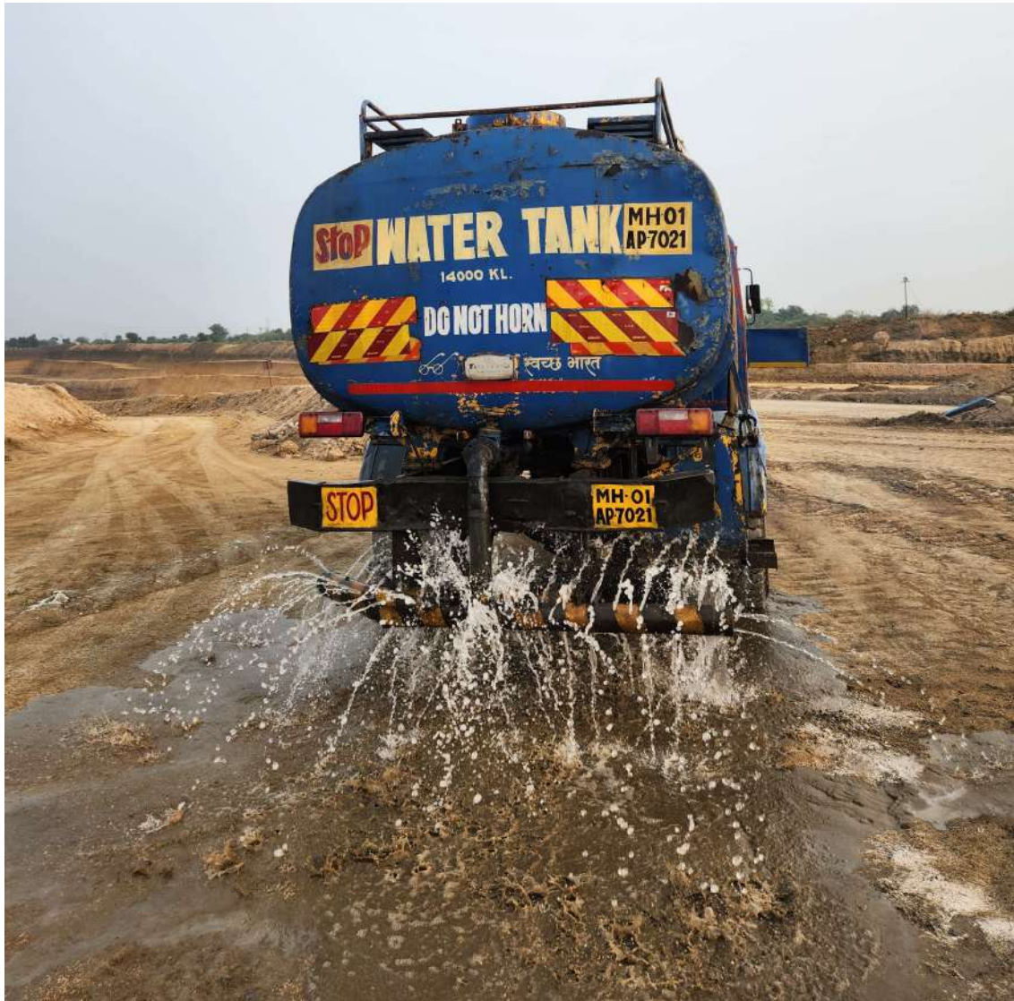
2. Water sprinkling on haul road near mine pit (12KL)
