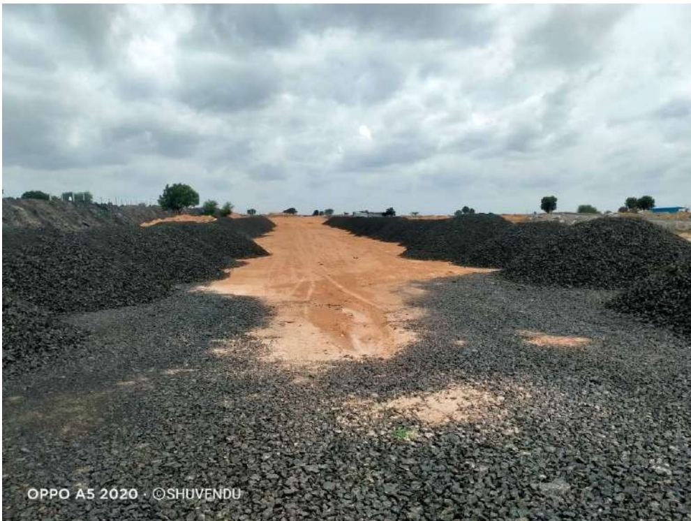
Transportation road work in progress
