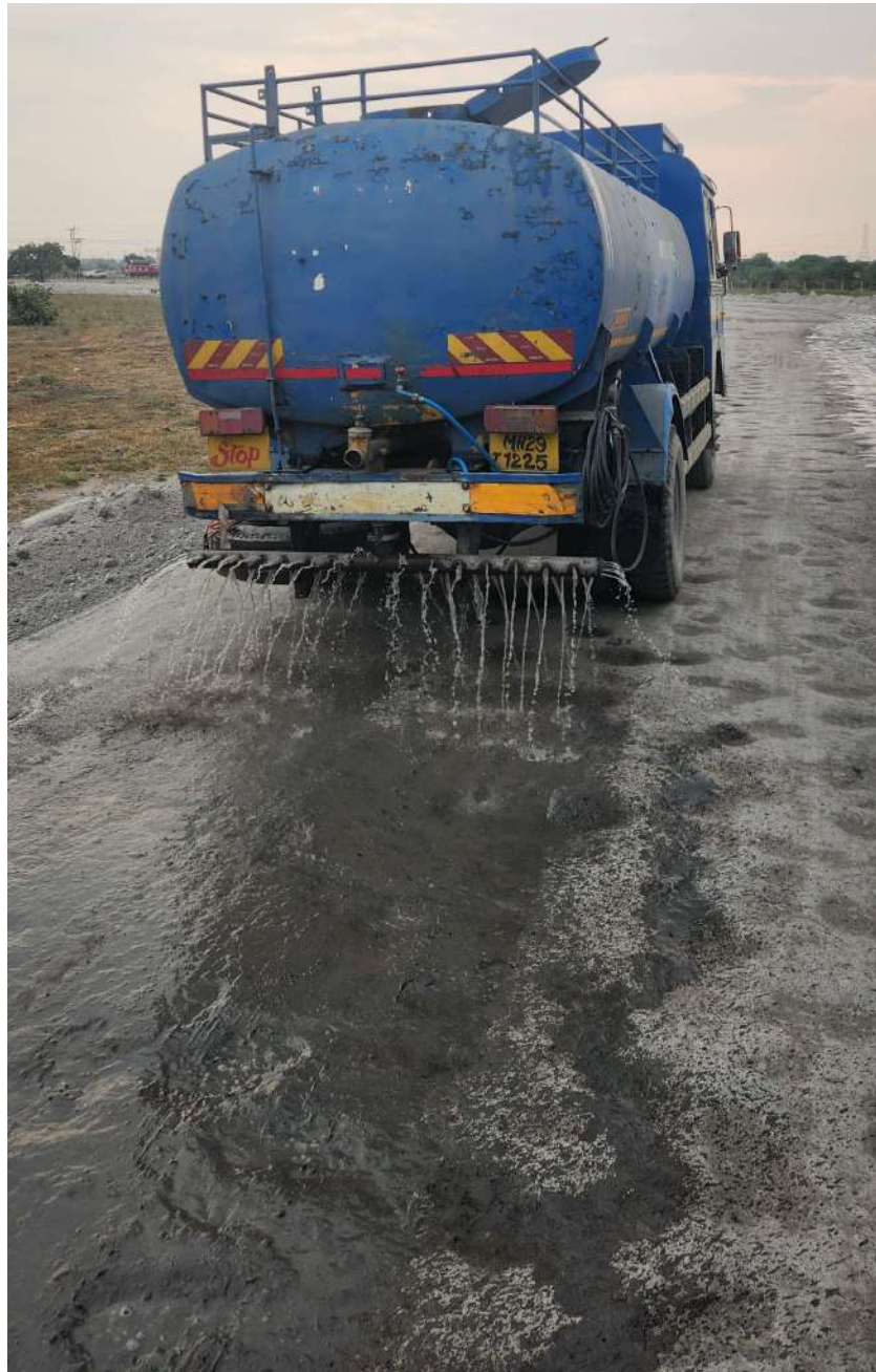
1. Water Sprinkling on transportation road (12KL)
