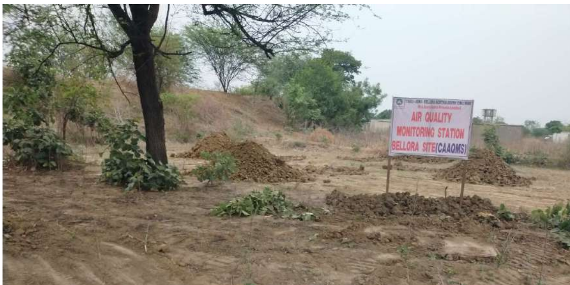
2. CAAQMS under installation
