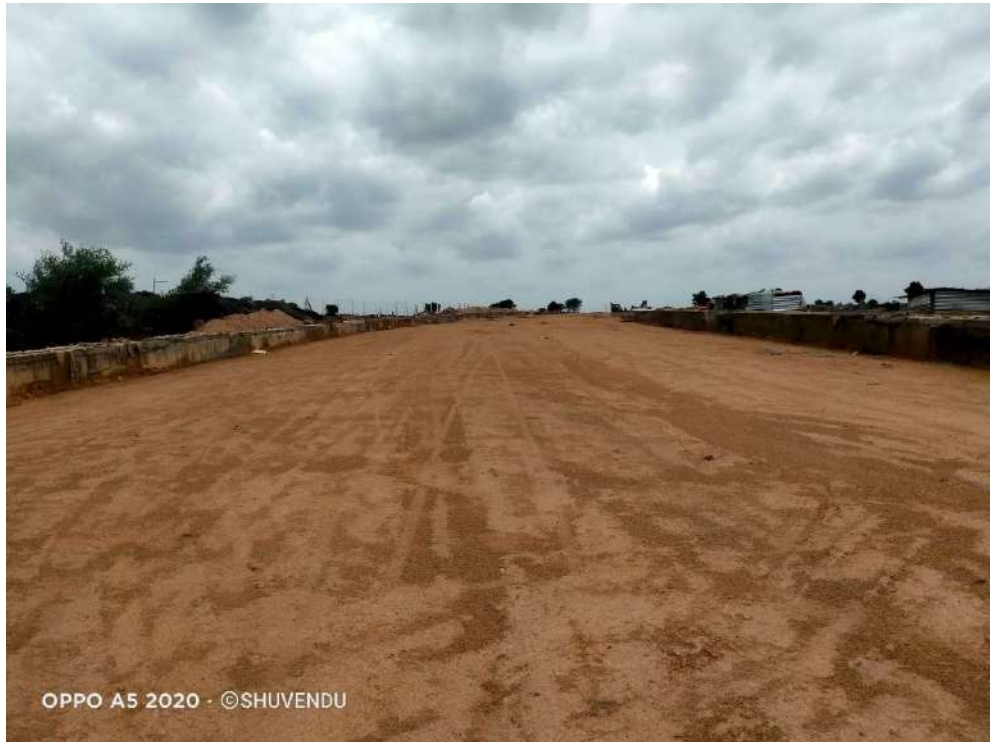
Transportation road work with side drains
