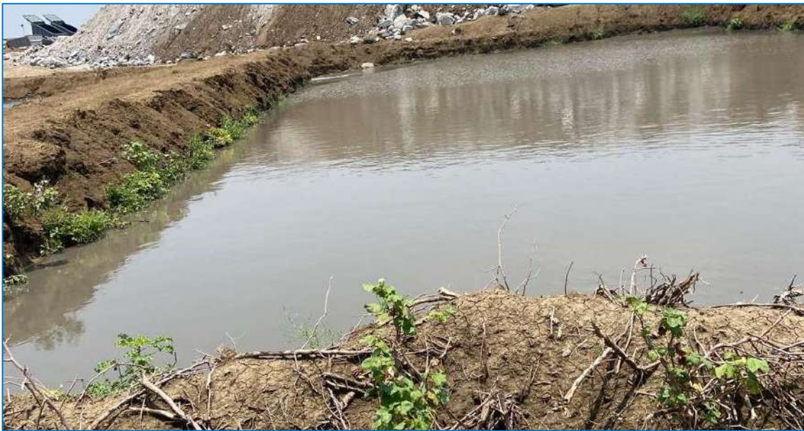
Series of Sedimentation tanks (3 no's)
